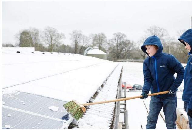
Figure 6: Snow removal with a broom. " Ramping up production at Balcombe's new " (CC BY 2.0) by 1010 Climate Action
