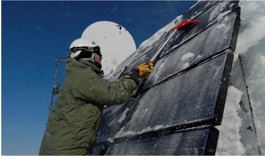
Figure 7: "Clears ice and snow from solar panels th" (CC BY-NC-ND 2.0) by U.S. Indo-Pacific Command
